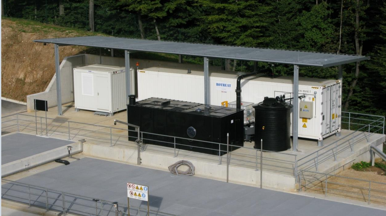
RO Novo Mesto, Slovenia 120 m 3 /d Leachate Treatment
