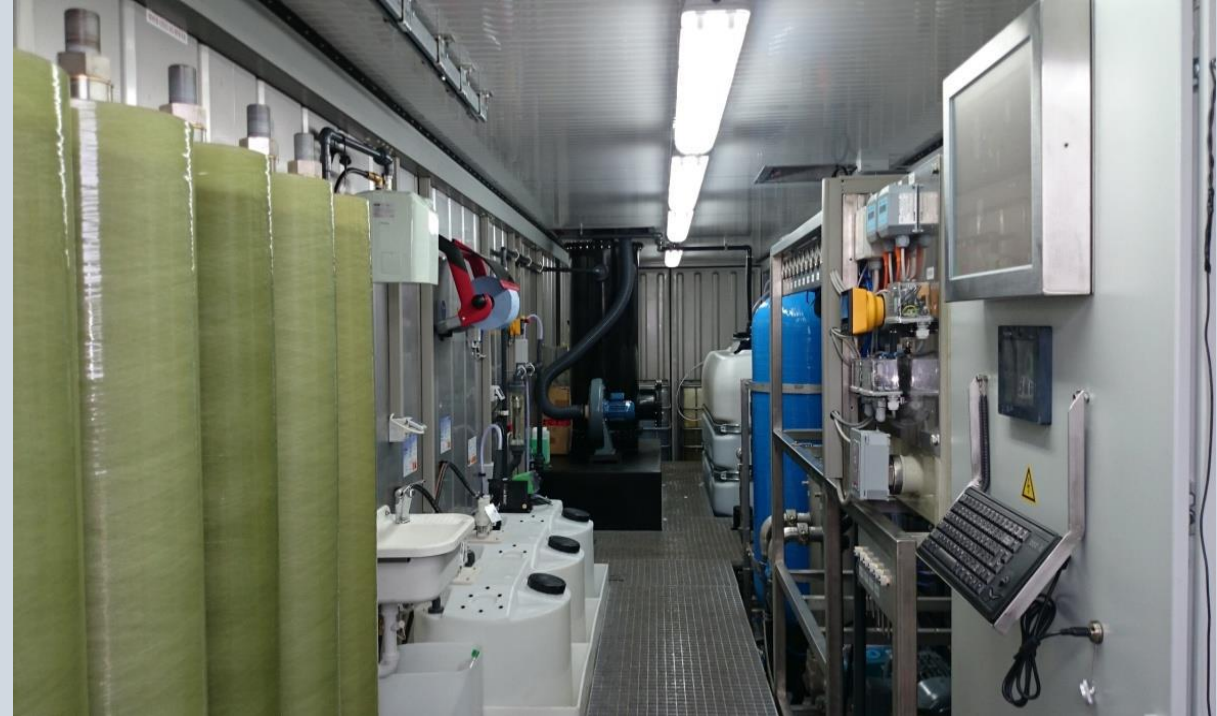
Bijeljina, Bosnia 35 m 3 /d Leachate Treatment
